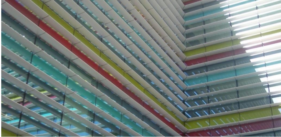
Figure 1. Fixed external installation of “passive” horizontal sunshade devices, as result of the aggregation of extruded aluminium shading devices (lenticular type) to façade curtains.
