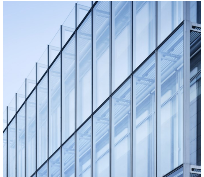
Fig. 10 Maurizio Varratta, iGuzzini Lab , Recanati. Assembly of the external screen, in the form of a totally or partially transparent façade, made up of monolithic tempered or double-glazed glass panes: this skin allows a ventilated cavity or as a buffer strip for thermal accumulation and insulation © Courtesy of Pichler Projects
